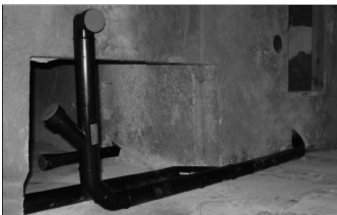
Illustration 6.2 Prefabricated pipe sections installed on site
